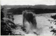
Fig. 5 – Destruction of the hydroelectric plant during the emptying of the penstock (August 1935)
