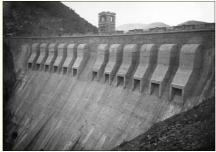
Fig. 2 – The Main Dam of Bric Zerbino showing the twelve dam siphons (O.E.G. photo, 1925)
